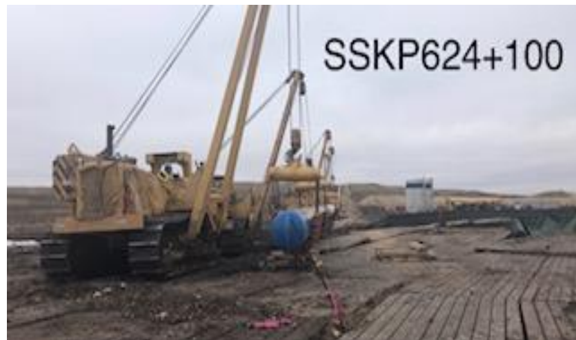
Prepping to pull drag section through Chapleau Lake
