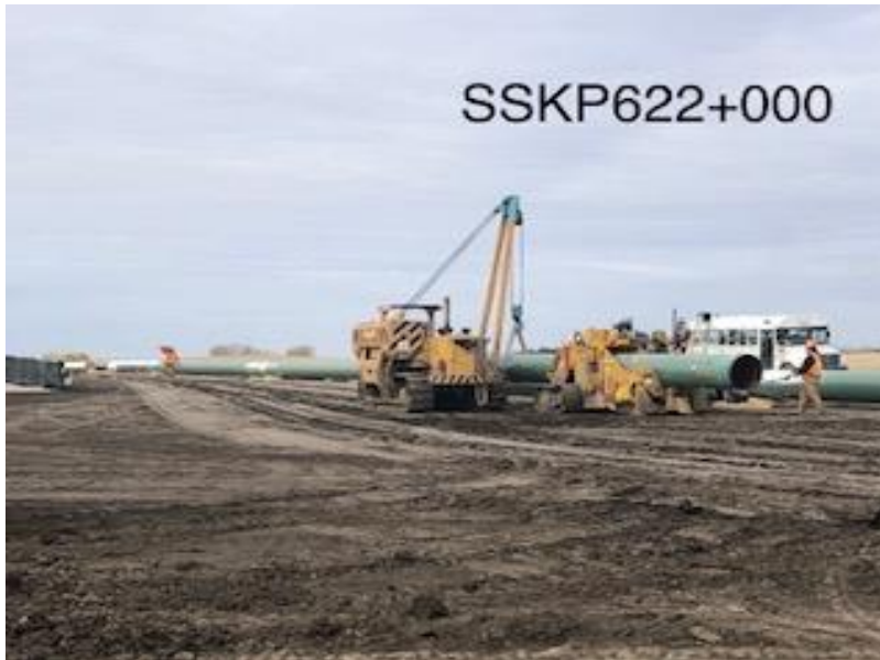
Bending crews reaching Native Prairie Zone SSKP622.28
