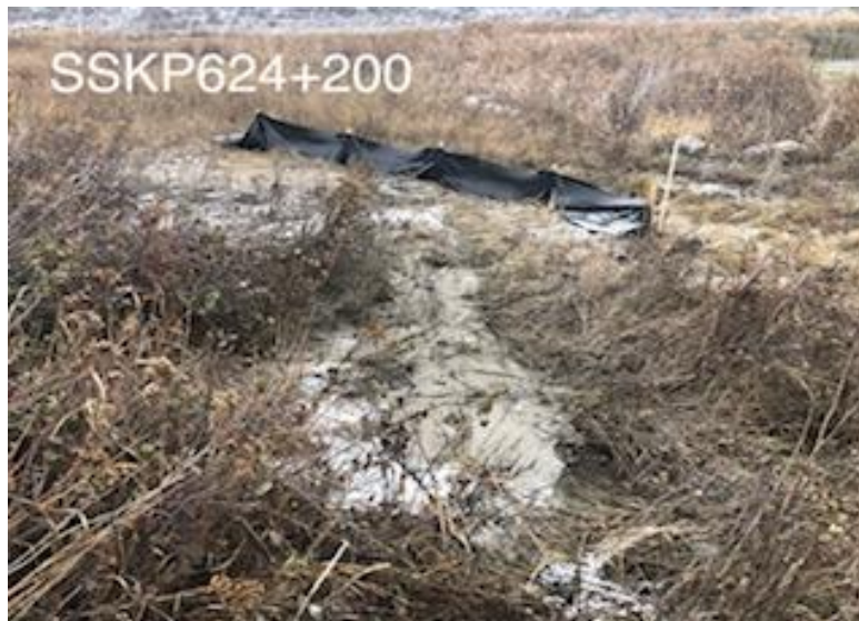
Frac-out west side of Chapleau Lake SK WC-68
