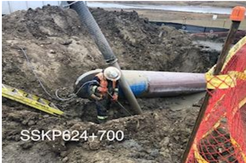
HDD pipe section reaching east side of chapleau
