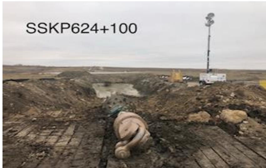
Prepping to pull the drag section at Chapleau Lake
