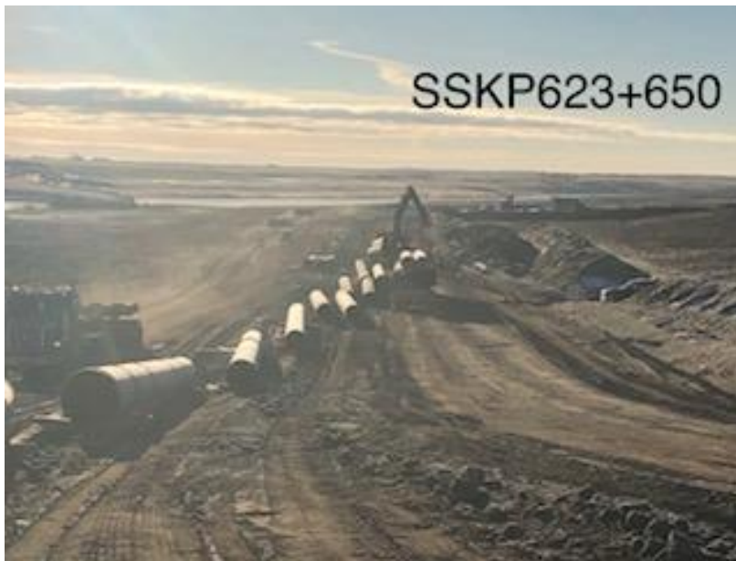
Stringing Crew West of Chapleau Lake
